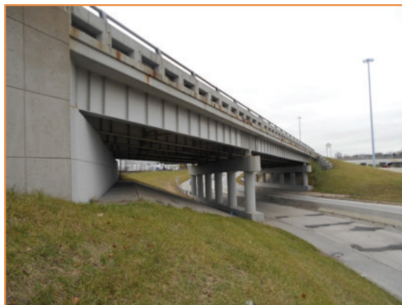
M-8/I-75 BRIDGE, DETROIT, MICHIGAN
