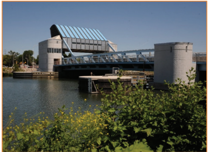
FORT STREET BRIDGE, DETROIT, MICHIGAN
